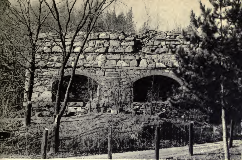
CEMENT KILN, WOODBRIDGE
